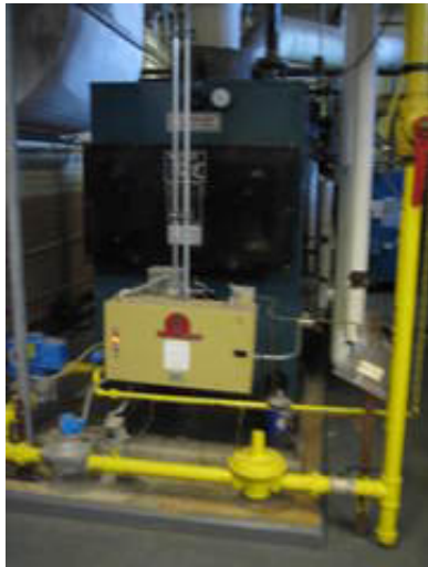
Gas fired steam boiler
