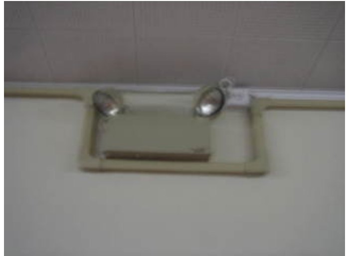
Self contained battery backup emergency lighting fixture
