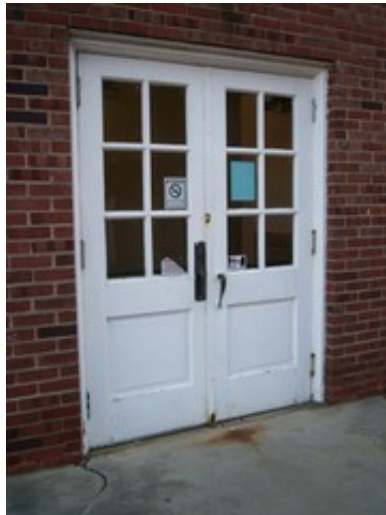
Wood entrance door
