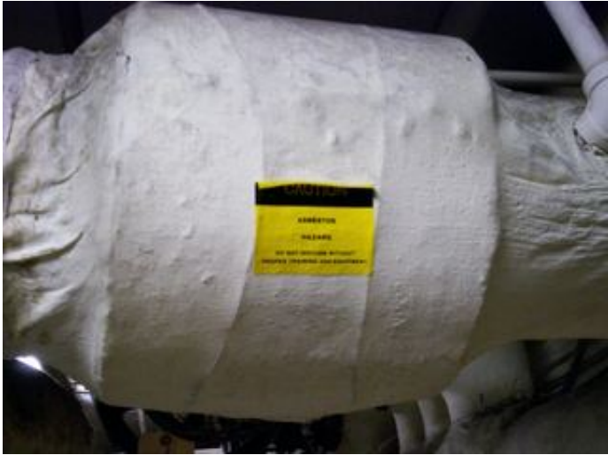
Asbestos label in mechanical room
