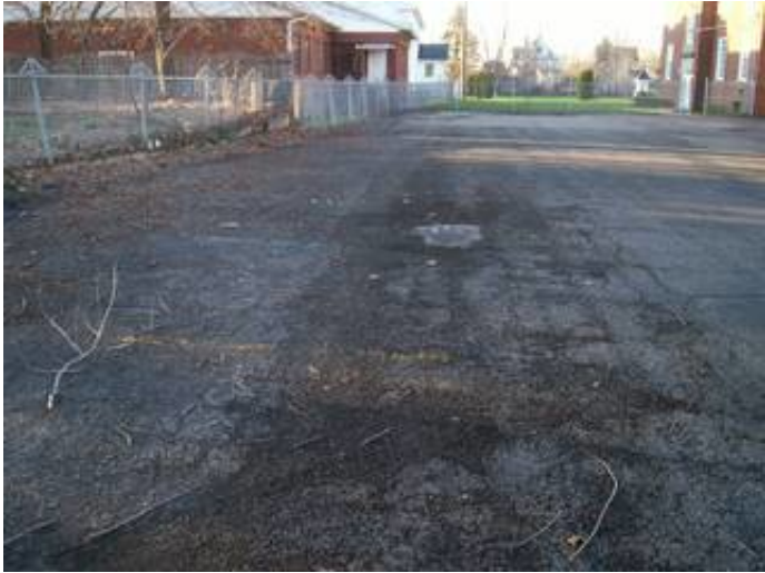
Asphalt pavement in poor condition
