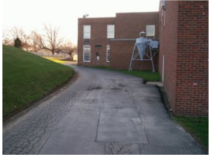
Asphalt pavement in poor condition
