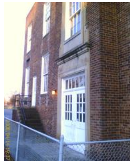
Typical exterior wall condition
