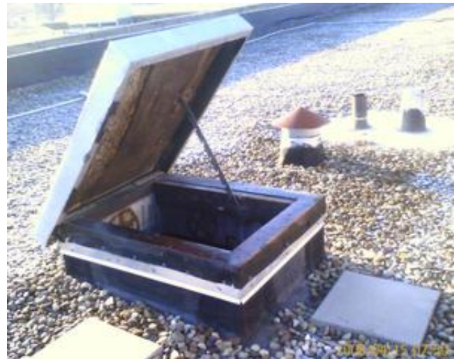
Typical roof hatch condition
