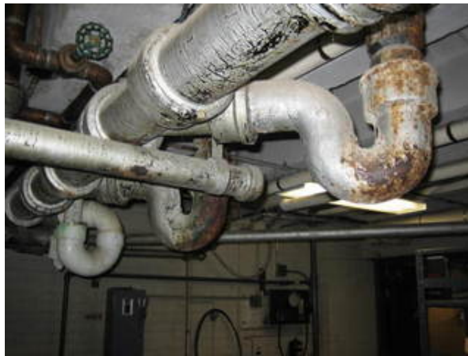
Cast-iron sanitary plumbing
