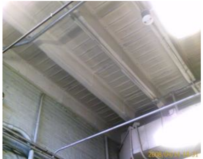
Typical cast-in-place concrete intermediate floor
