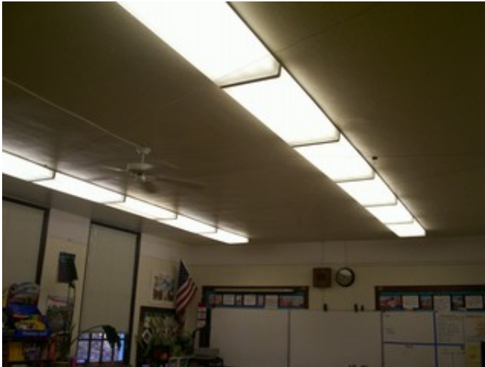
Typical classroom lighting
