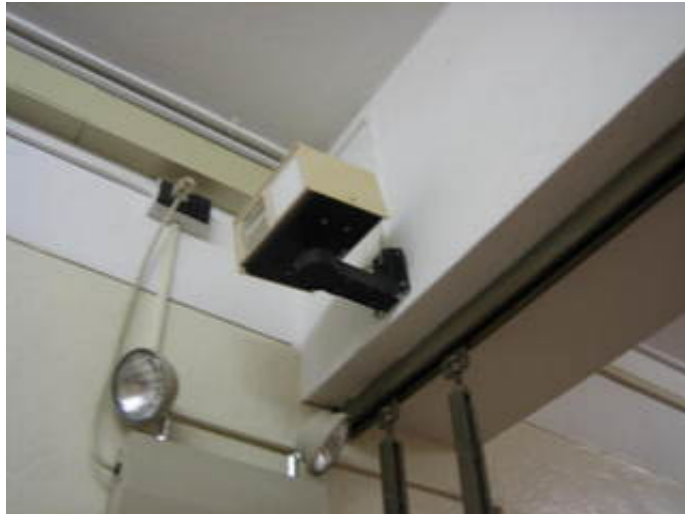
Corridor mounted motion sensor
