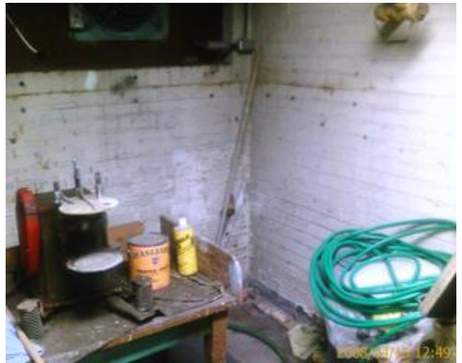
Typical masonry foundation wall
