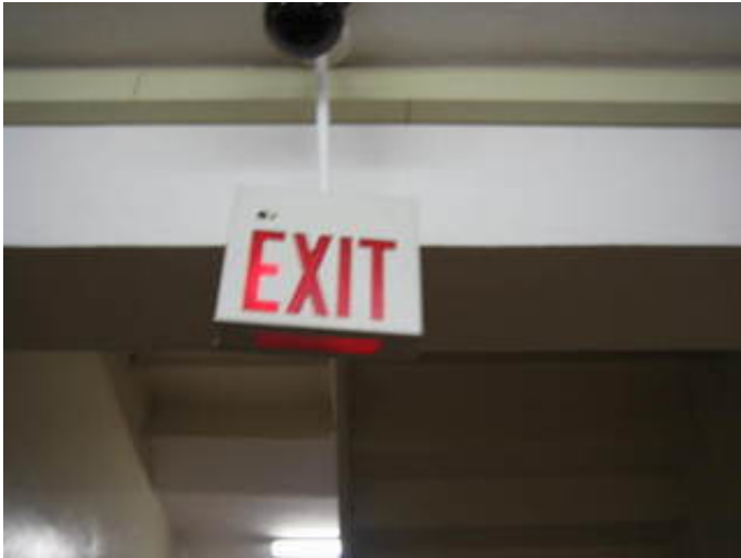
Corridor mounted exit signage
