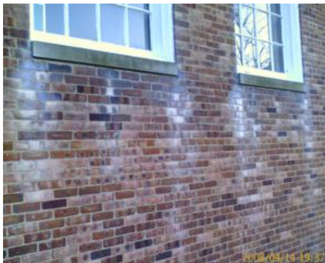
Typical exterior wall condition
