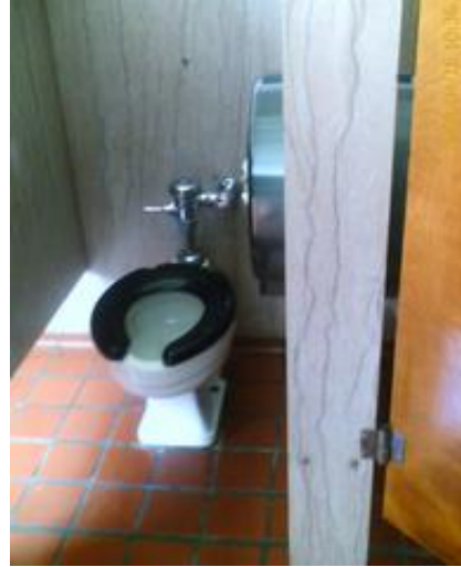
Typical toilet condition
