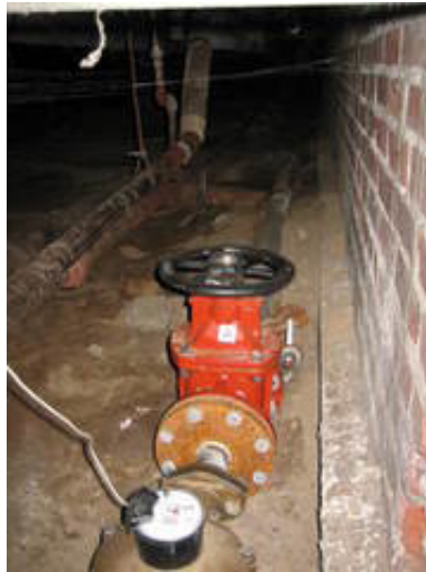
Water service entry
