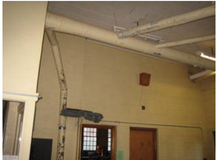
Wood shop dust collection system
