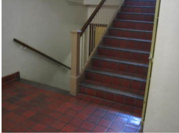
Unenclosed egress stair
