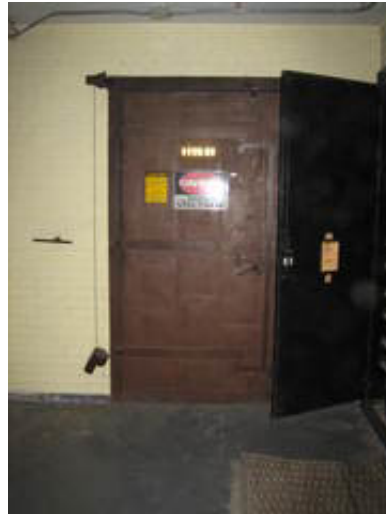
Transformer vault in basement
