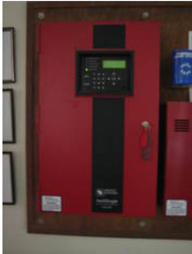
Security panel in administration area
