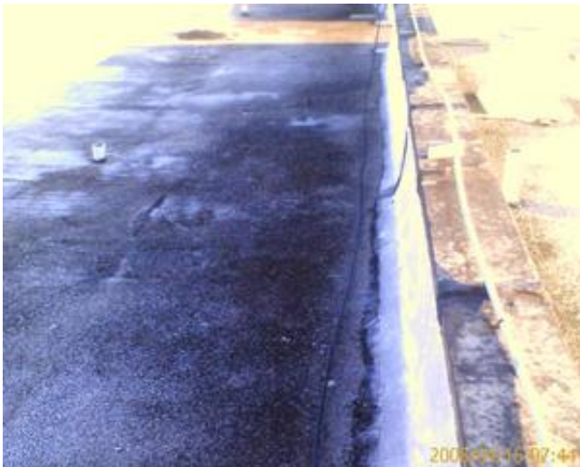
Typical roofing condition
