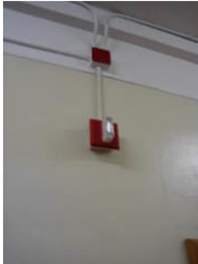
Corridor mounted horn/strobe device
