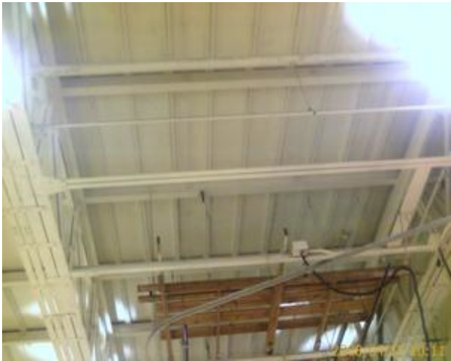
Typical wood roof deck
