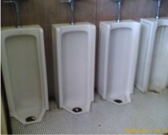
Typical floor mounted urinal
