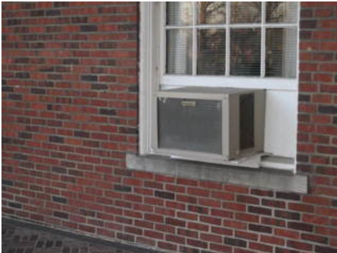
Window air conditioning unit
